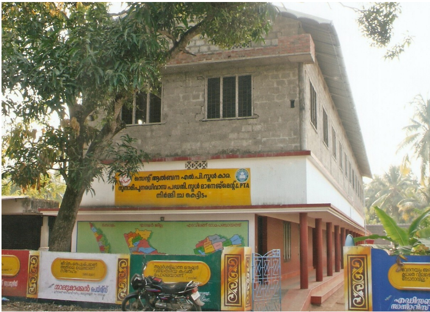
School reconstruction in progress
